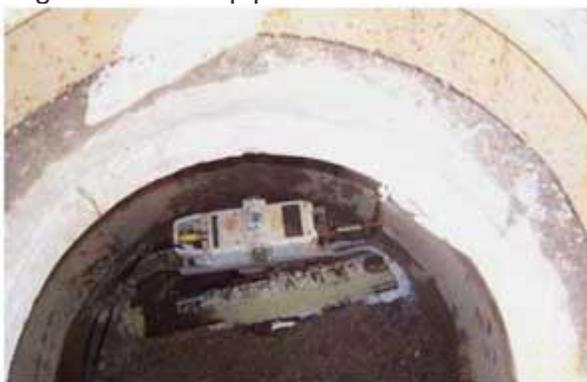
DDS FLO-DAR Sensor monitoring flow in 8" Sewer Line
