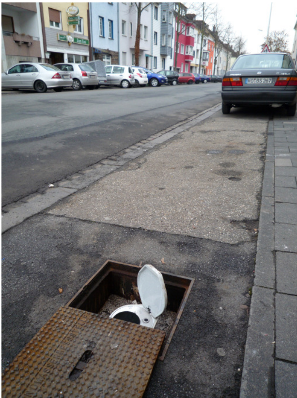
Urban measurement network – groundwater monitoring in the city with OTT Orpheus Mini
