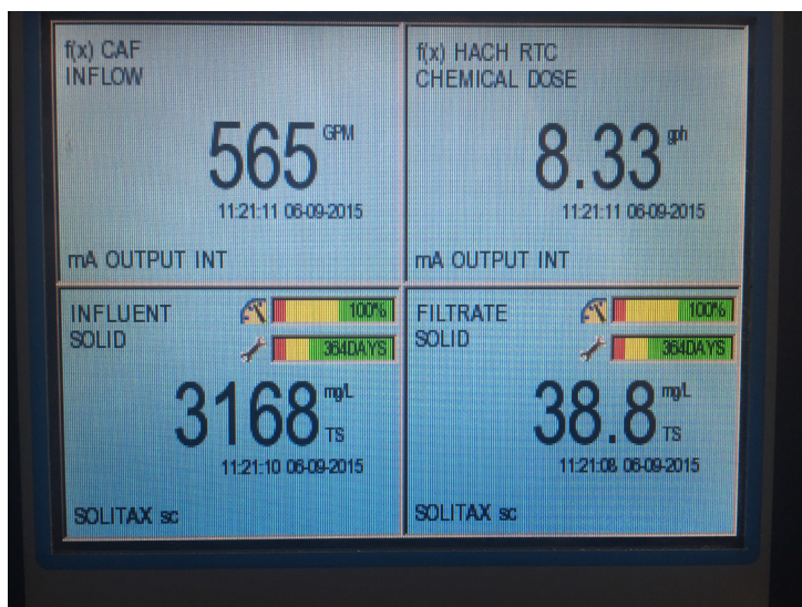
Figure 2: Real-time control automatically balances TSS requirements with pH level limits, eliminating the need for manual measurement and dosing.
