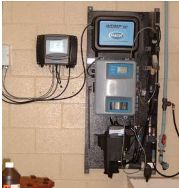
The Hach Water Distribution Monitoring Panel (WDMPsc) is a compact panel fitted with four analyzers to monitor free or total chlorine, turbidity, pH, conductivity, temperature and sample pressure.
